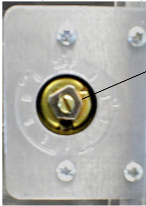
Fig 1 Temperature Control Adjustment. (Arrow shows location of adjustment screw)
